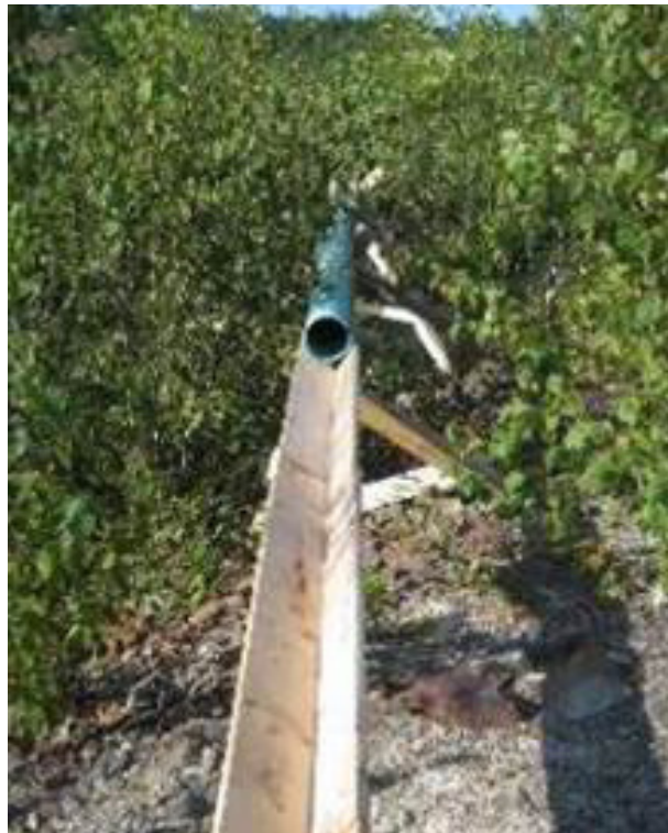
A high pressure hose, contained in secondary containment, and draining naturally downhill, ensured that treated water was not contaminated during drilling at the East Kemptville Project.
