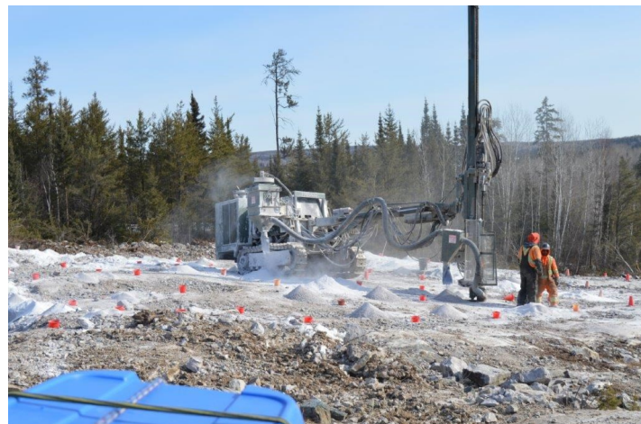
Blasting caps being placed Separation Rapids
