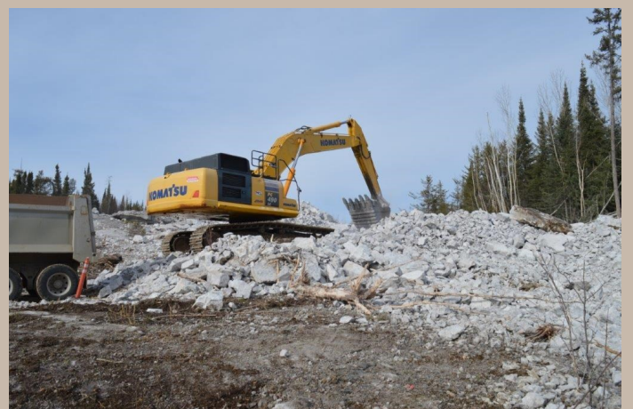
Work during Separation Rapids Bulk Sample
